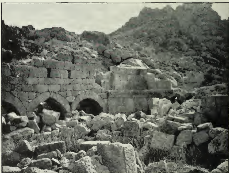
FIG. 146.—No. 34, interior from S.-W.
